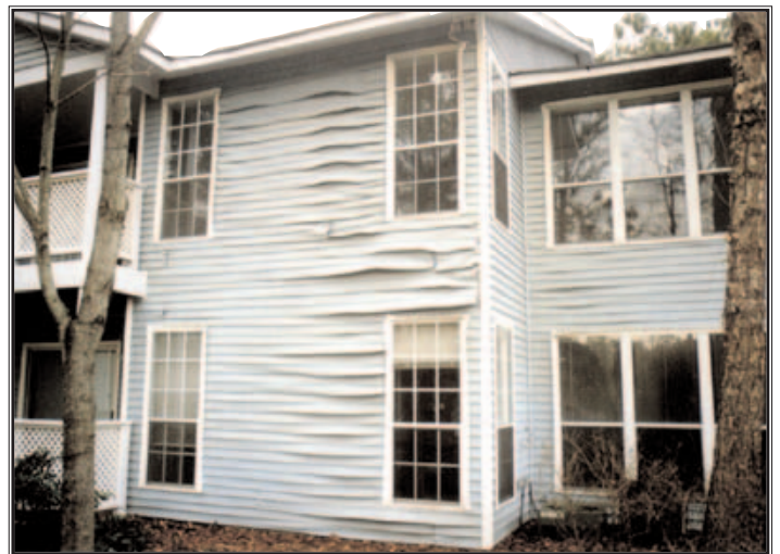
Vinyl siding melted from heat generated by a burning building 50 feet away
