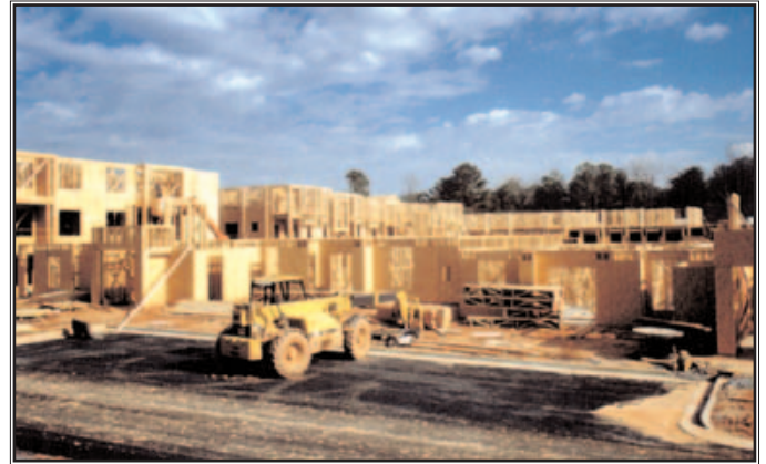
Apartments under construction illustrate why one hour combustible separations do not confine fires. The one-hour separations themselves add fuel to the fire
