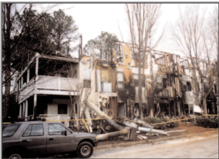
Fire department response time -- 3 minutes. Ten families homeless. Building -- total loss.
