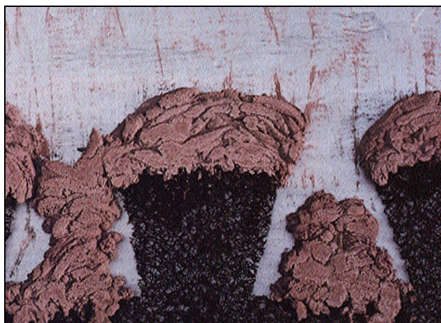
Figure 5. A new type of nylon fiber mesh is said to distribute mortar buildup in a way that creates clear paths for water to drain through weep holes.
