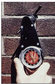
Expansion anchors for pinning brick have two expansion sleeves, one for the backup and one for the facade. First the inside sleeve usually is installed (top) then torqued (bottom). Then the outside sleeve is installed and torqued.
