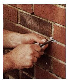
Adhesive anchors are installed by filling a screen tube with adhesive (top), inserting the tube in a clean, drilled hole (middle), then inserting a steel rod inside the screen (bottom). Inserting the rod pushes the adhesive through the screen into the masonry, bonding the two together. million, this was still less expensive than closing the warehouse, demolishing the walls, and rebuilding them.
