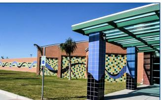
Glazed brick can be used as loadbearing, cavity or veneer walls. The fired clay material can provide the durability and longevity that is required for schools, municipal buildings, libraries, museums, and art centers, for example.
