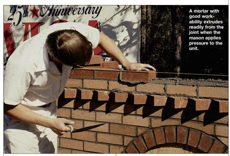
include increased workability and water retentivity, and the ability to deform slowly in the hardened state, thereby accommodating some structural movement.
