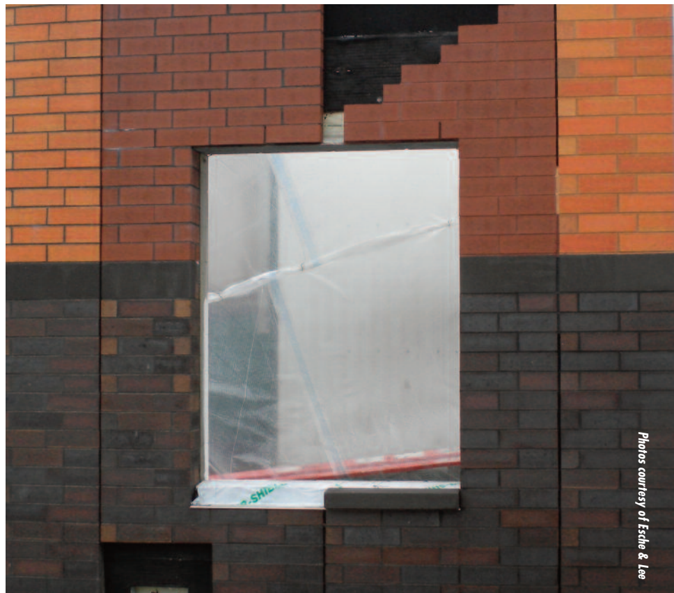
A mock-up panel, complete with openings and sills, represents what the owner and architect expect in the final building. It will also allow the design and construction teams to identify and allow for the resolution of issues before construction begins.
