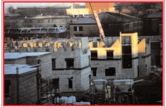
NOTE HOW THE FLOORS ARE COMPARTMENTALIZED WITH THE USE OF HOLLOW-CORE PRECAST PLANKS
