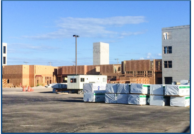
3 CMU Towers are built early in the construction phase.
