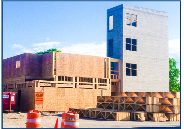
CMU Towers aid workers as they build.
