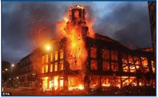
A CMU stair tower in this building could save lives.
