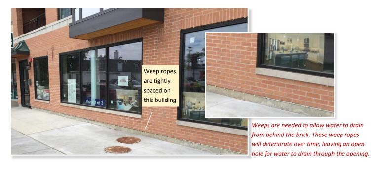
The Brick Industry Association <u>Tek Note #7</u> – **Water Penetration Resistance Design and Detailing**, actually recommends leaving an <u>open head joint</u> formed by leaving mortar out of a head joint. These openings need to be at least 2" high. It further explains that non-corrosive metal, mesh or plastic screens can be installed in the open head joints. Spacing of these weeps are recommended at 24" on center.
