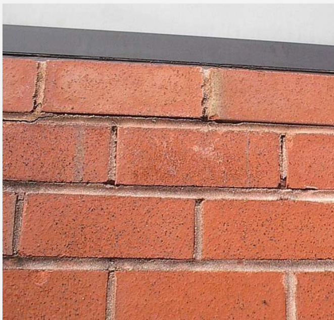
Mortar Joints in Need of Repointing
