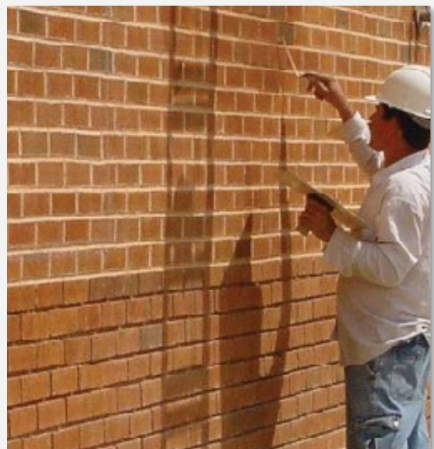
Repointing Mortar Joints
