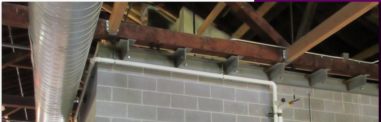
Level 4: Truss Reinforcement - 2016
