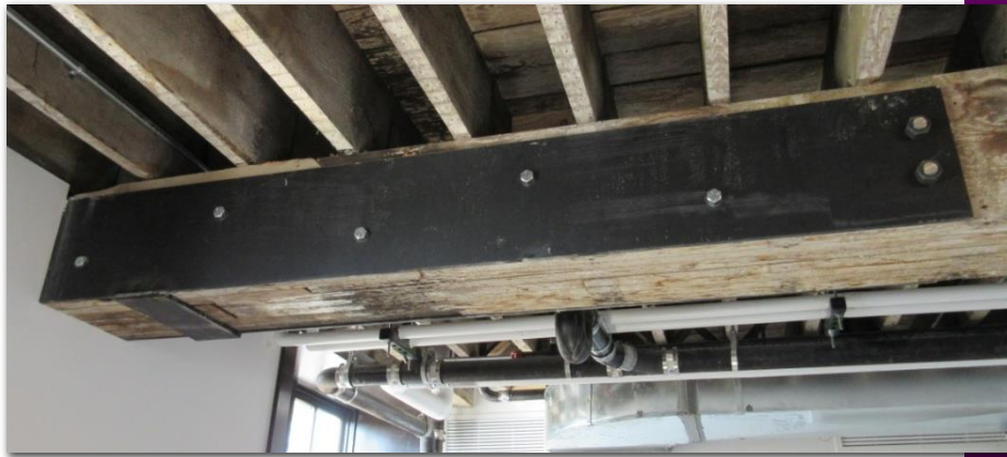
Level: 1 Beam Reinforcement - 2016
