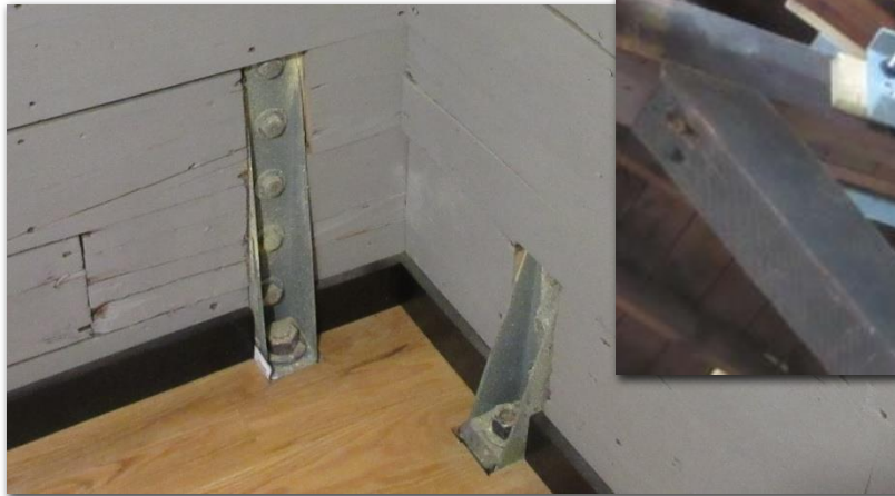
Level 2: Corner Reinforcement - 2016
