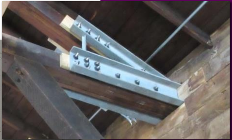
Level 4: Truss Bearing Reinforcement - 2016
