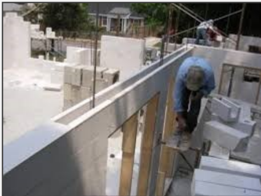
Concrete block lintel
