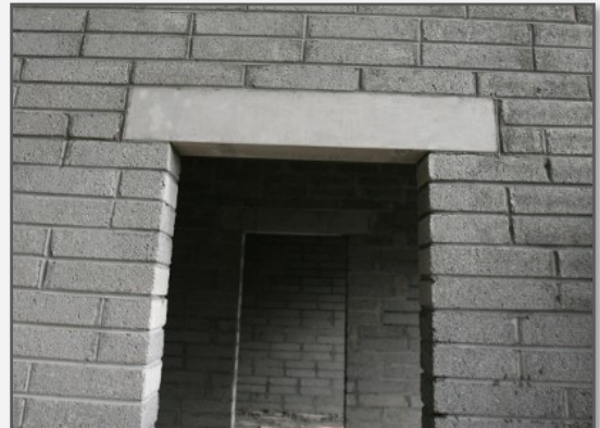
Reinforced concrete lintel
