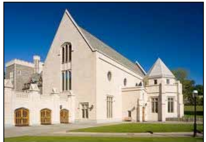
Figure 1—Dining Hall Whitman College, Yale University, with Diaphragm Walls Constructed in 2007
