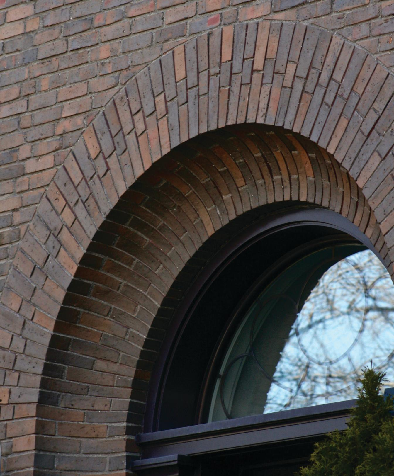
Brent Schmitt of Bricks Inc. calls it “a 3D arch.” It’s a fitting name. Each brick in the arch is perfectly shaped in three dimensions to perfectly fit in its place. As the bricks on the front edge taper from top to bottom, they must also taper backwards to fit into the scoop below the arch.
