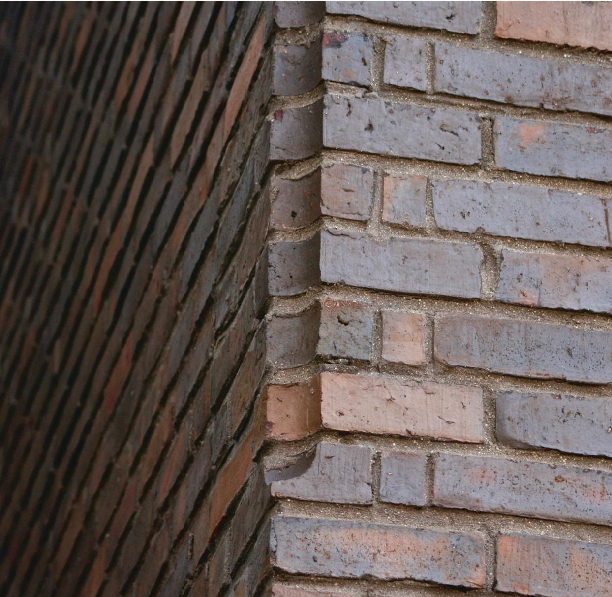
The next step in reducing the scale of the house was to reduce the perception of the vertical mass. Sellars designed the house as a “two story volume, with a smaller one on top.” The top story is divided from the rest by a sort of false cornice: scooped bricks flare out into several courses of stretchers topped with a limestone band, upon which rests the third story.
