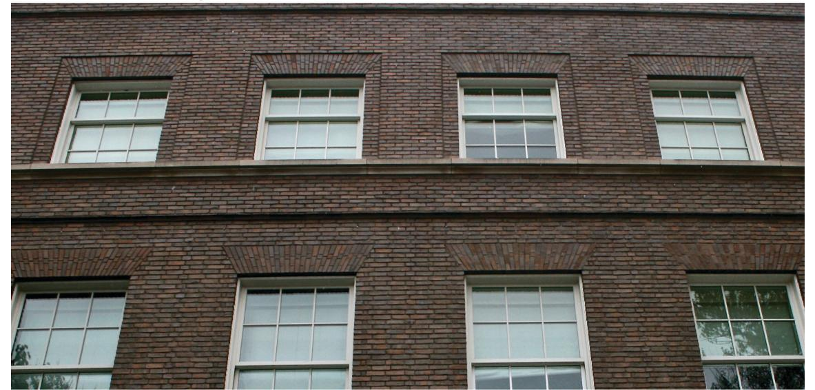
Between the 1/2 bricks, scooped bricks, and even small 1/3 bricks (used around the windows as a nod to brick firestops used in the Georgian townhomes of South London), Bricks Inc. sourced over 20 custom hand-molded shapes for 1853 N Burling.
