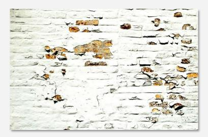
There is an alternative to painting brick. This alternative is staining the brick. Staining is a process that penetrates the surface pore structure of the brick or masonry making a bond with the unit. Paint is a surface coating that mask the texture not making the chemical bond with the unit. In painting since there is no good bond with the unit, water can come into the air space between, allowing water to freeze and pop paint off the surface.
