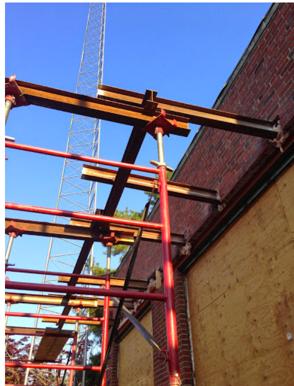
Figure 2: Temporary Needle Shoring Source: Superior Scaffold Services
