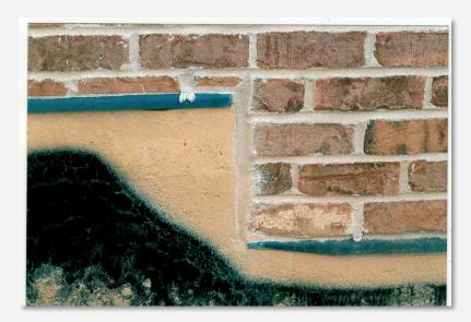
If the step flashing is installed in accordance to figure 1, proper water drainage will be achieved and water penetration to the interior will be eliminated.
