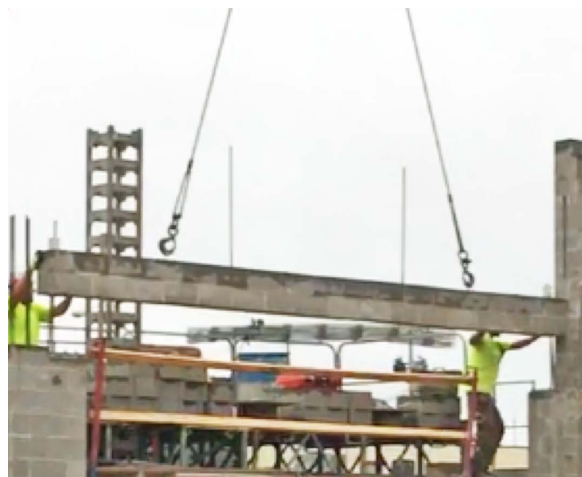
Figure 1: Prefabricated Masonry Lintel
