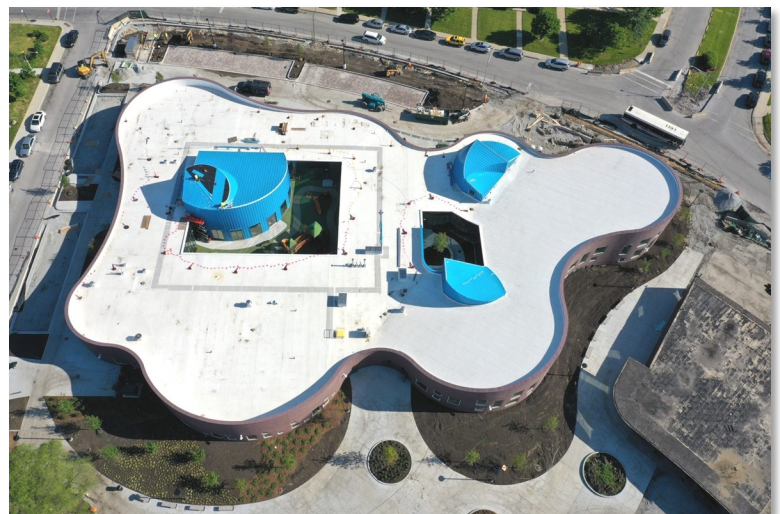
Robert Klein, Superintendent of ALL Construction Group stated that GPS was used to calculate the radius and rake of the concave and convex walls, and it was used to establish points for radius at windows and entry points.
