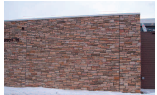
Picture 2. Adhered veneer with movement joints properly installed. By code, these movement joints must be shown on the drawings.
