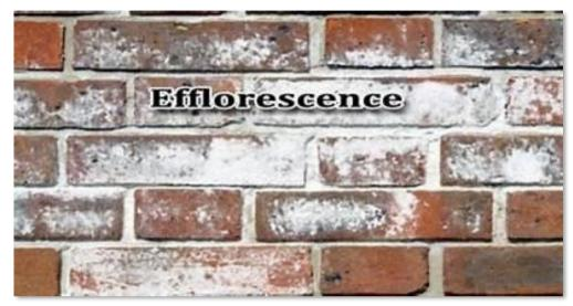
Many buildings at some point in their history exhibit some form of efflorescence. What is efflorescence? Efflorescence is a white chalky substance that often occurs on the surface of a masonry wall and it is comprised of water-soluble salts. When soluble salts are dissolved in water, this becomes a salt solution. The salt solution then moves to the surface of the masonry wall where the water evaporates and leaves the salts on the surface, that is efflorescence.
