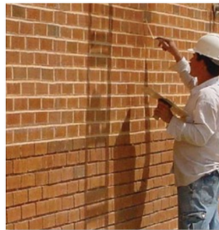
Repointing Mortar Joints
