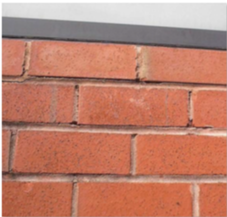
Mortar Joints in Need of Repointing
