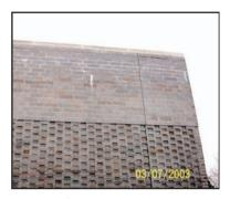
**My Bank:**(Note the efflorescence, and the flush limestone cap- it should have had 1 1/2"projection or a drip edge and flashing under the cap)
